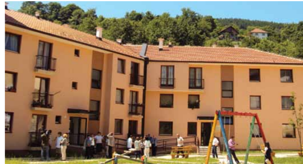
A social and cultural center in Bosnia and Herzegovina, funded by the Zayed Foundation. (Source: Zayed Foundation)
