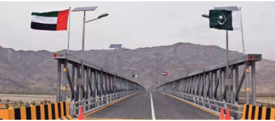
The Sheikh Khalifa Bin Zayed Bridge over the Swat Valley in Pakistan. (Source: UAE Pakistan Assistance Project)
