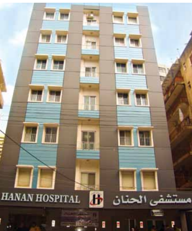
Al Hanan Hospital in Tripoli, Lebanon, funded by the Zayed Foundation (Source: Zayed Foundation)
