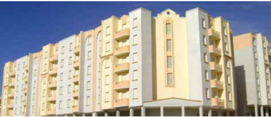
The Satif residential housing project in Algeria, funded by the Abu Dhabi Fund for Development. (Source: ADFD)
