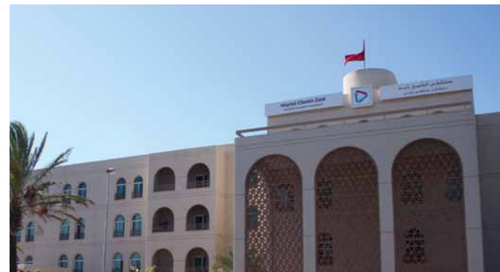
The Sheikh Zayed Medical Hospital in Rabat, Morocco, supported by the Abu Dhabi Fund for Development (Source: Prima Media)
