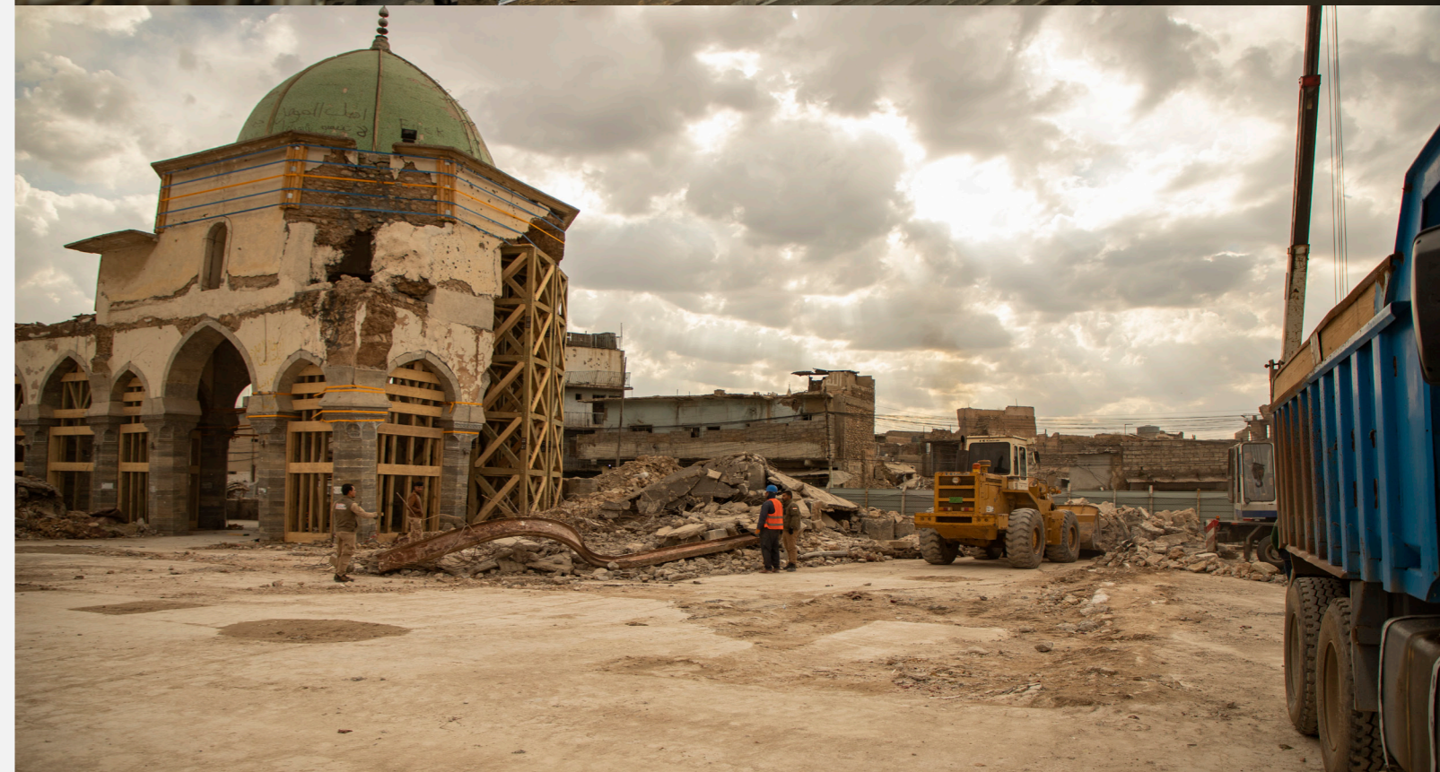
Renovation of the ancient cultural site Al-Nuri Mosque. Source: UAE Ministry of Culture and Knowledge Development (MCKD)
