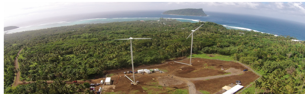
Wind farm project constructed in the Upolu island in Samoa, which is home to nearly 75 percent of the population. The wind farm project supplies 1,500 megawatt-hours of power per year. Source: MASDAR
