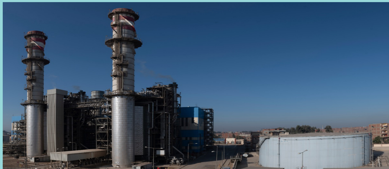
The power station has a capacity of 750 MW and is linked to the national grid on a 220-kilovolt transmission line. The power station served the large urban and agricultural bloc of Benha, the capital of the Qalubia Governorate in the East Delta. Source: Abu Dhabi Fund for Development (ADFD)
