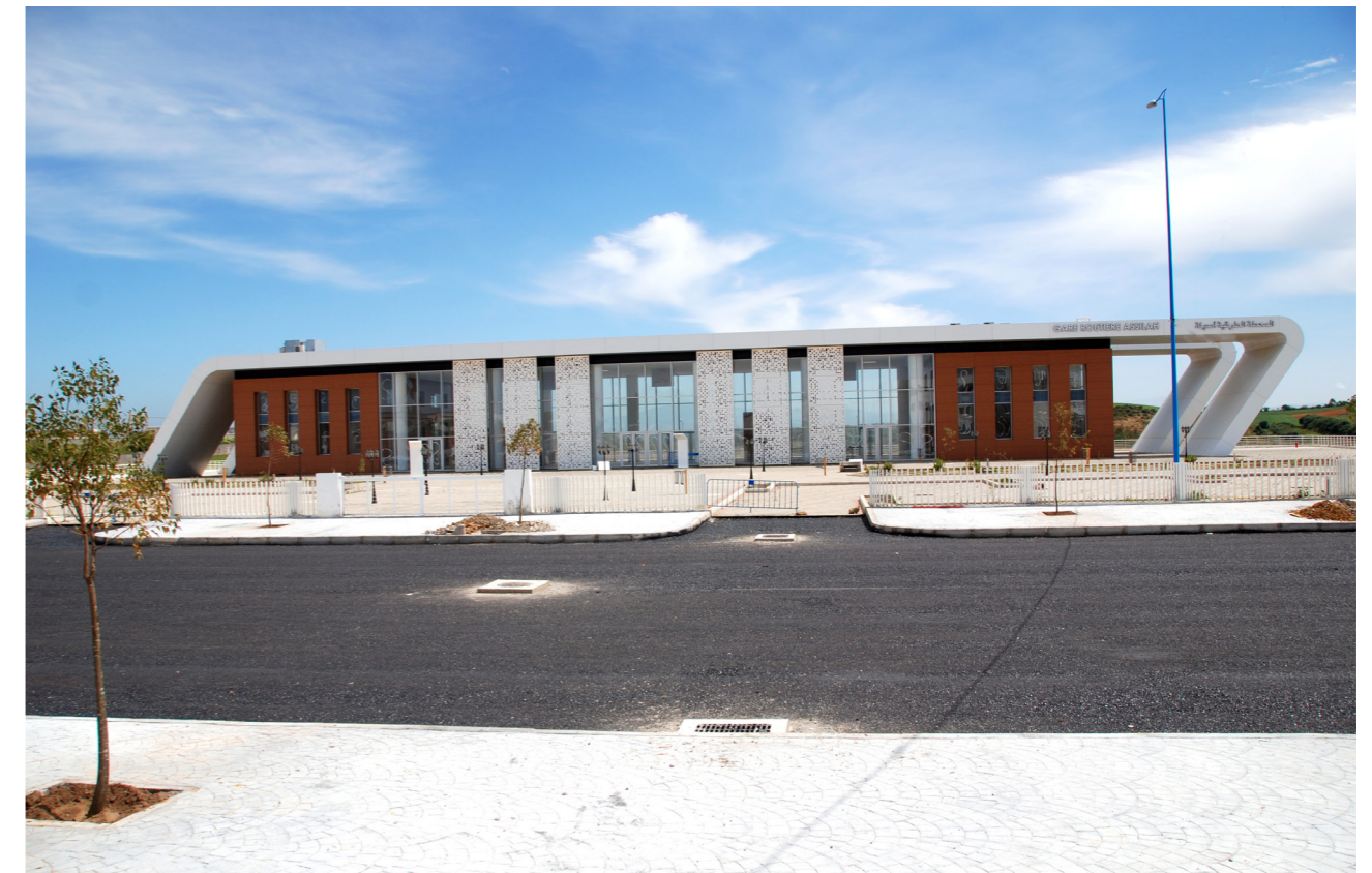
Road station funded by Abu Dhabi Fund for Development in Asilah town in Morocco. Source: Abu Dhabi Fund for Development (ADFD)
