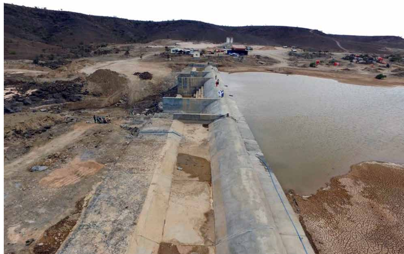
11-metre-high concrete dam with a capacity of 350,000 cubic metres saves 650,000 gallons of water daily during the dry season in the Hargeisa area in Somalia.
